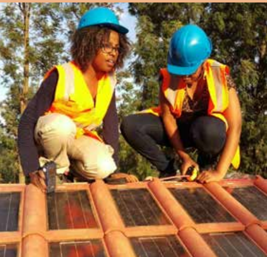
A team installs solar powered roofing tiles on a house. Innovation is key to achieving green growth. ©Climate Innovation Centre
